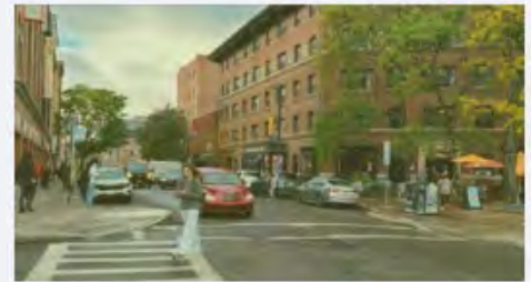
The planned redesign and reconstruction of College Avenue's 400 block (image) would tend to the infrastructure needs of that one stretch, but a similar effort seems necessary for the district as a whole.
